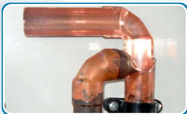
Brazing with Inert Gas Shield
